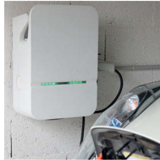
1 Charging station Electric energy brings you everywhere. Charge your car while you are working thanks to dedicated charging stations by Hager.
